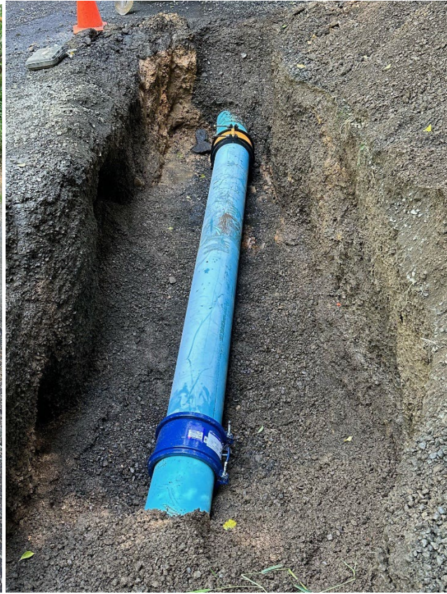
11-foot replacement pipe, with repair couplings:
