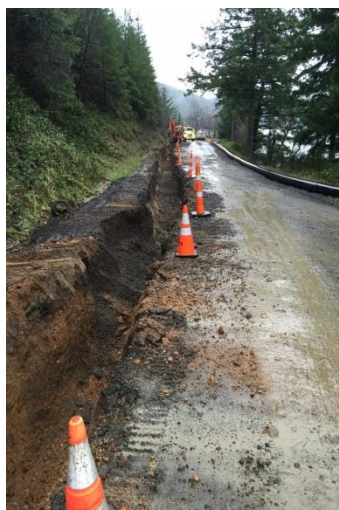
New fused 14-inch HDPE Pipe:
