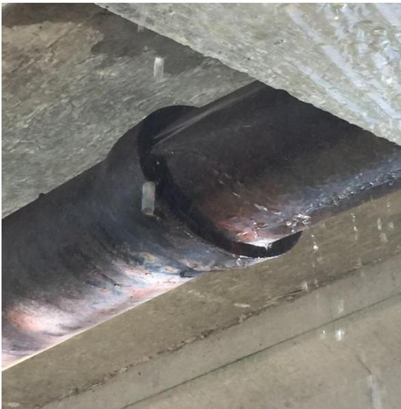
*Leaking 12-inch bell joint:*
