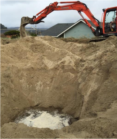
Lowering Sand Dune for safe Access:
