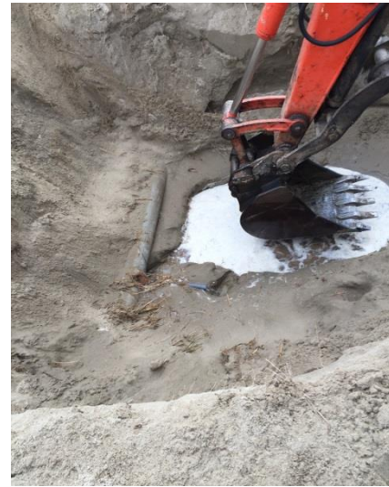
Exposing Pipe 20-feet deep:
