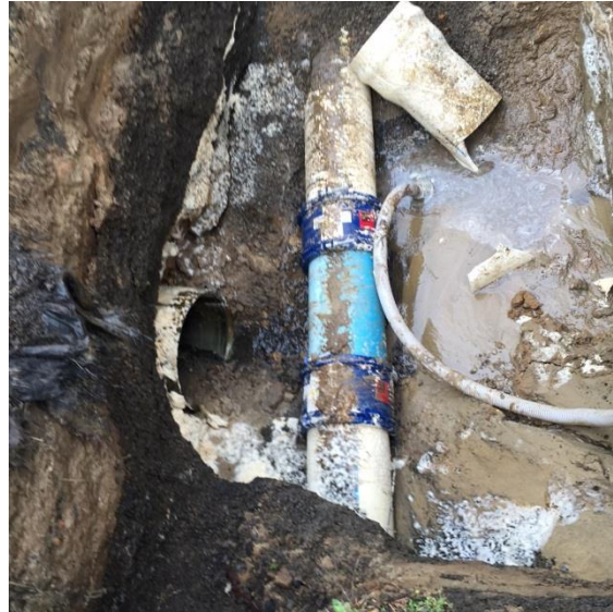
Completed Repair with Pipe Casing to the Left:
