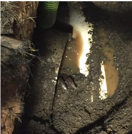
Boring Head into the Water Line:
